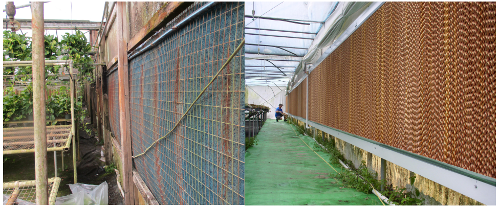
(Left) Conventional hog-hair evaporative cooling pad with no water recycling system. (Right) New, efficient cellulose evaporative cooling pad with water recycling system.
